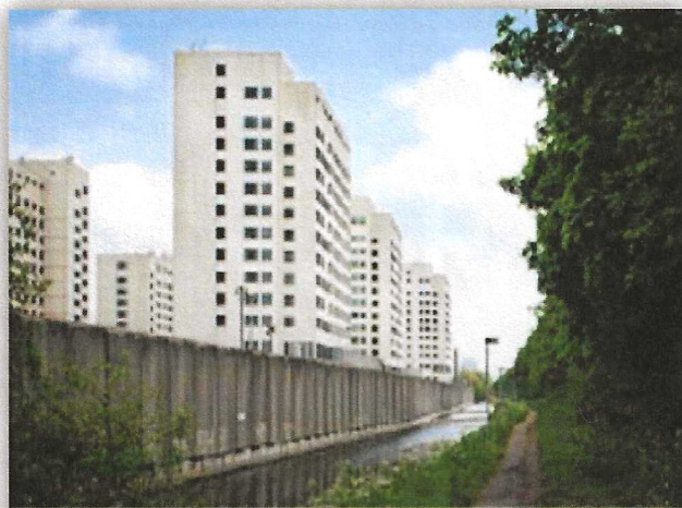
Figure 6 Correctional facility Over-Amstel Netherlands ( High-Rise Layout )
